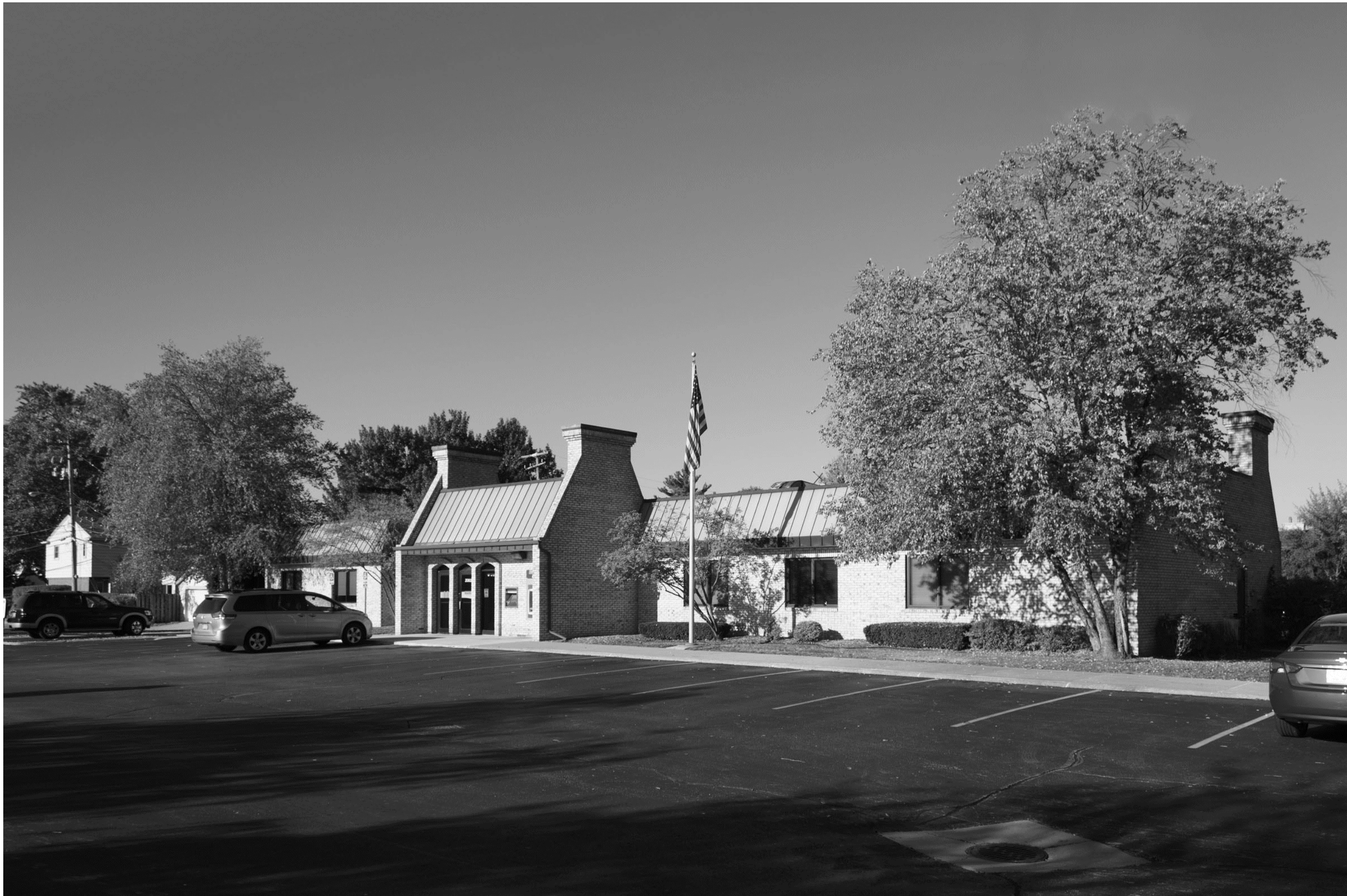
1 FRONT FACADE - EXISTING
