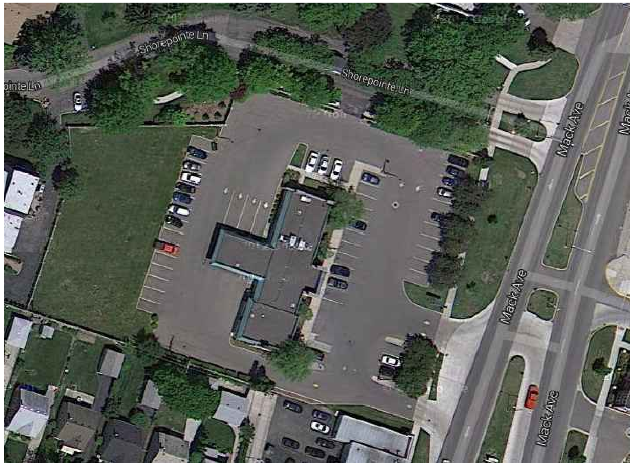
EXISTING AERIAL VIEW
